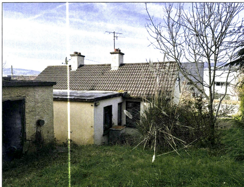
Figure 3: View of rear of dwelling showing sloping ground, with existing shed raised above the level of the existing dwelling and extension (source: daft.ie)
